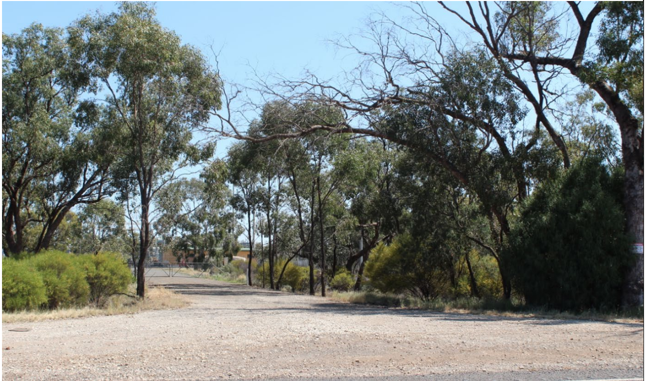
Figure 3-33 Viewpoint 6 from the Kidman Way looking at the Essential Energy zone substation (NGH, 2023)
