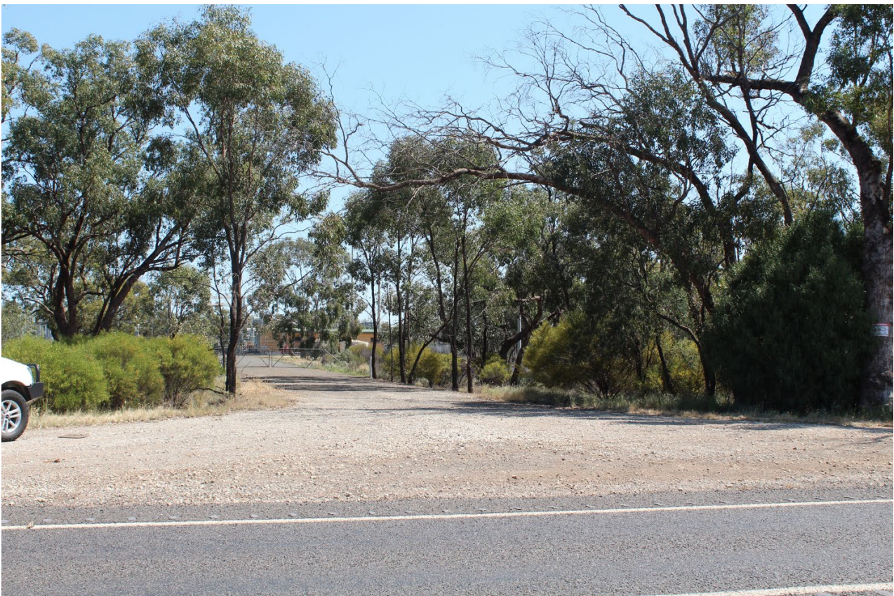
Figure 3-12 View of Essential Energy substation from the Kidman Way
