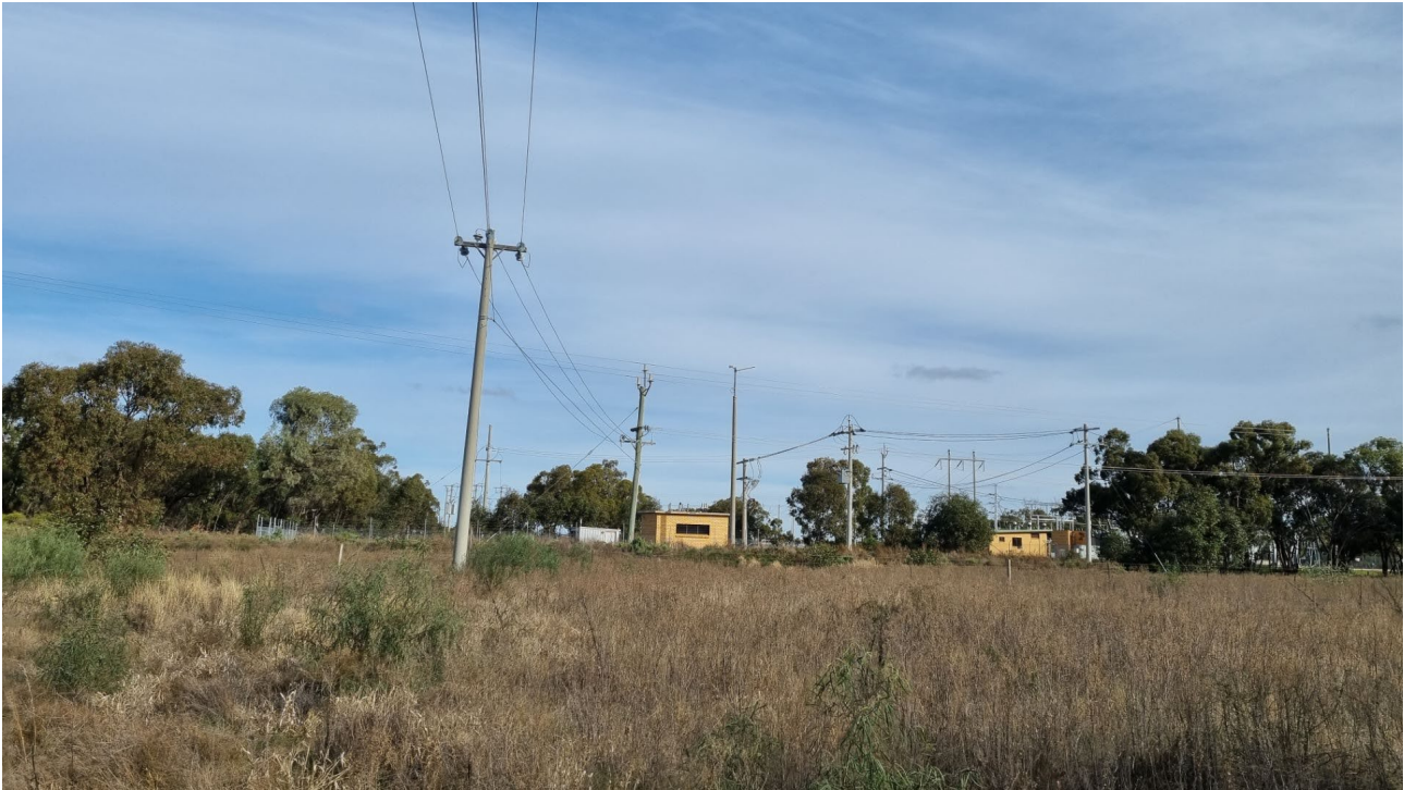
Figure 3-7 View east to neighbouring Essential Energy zone substation
